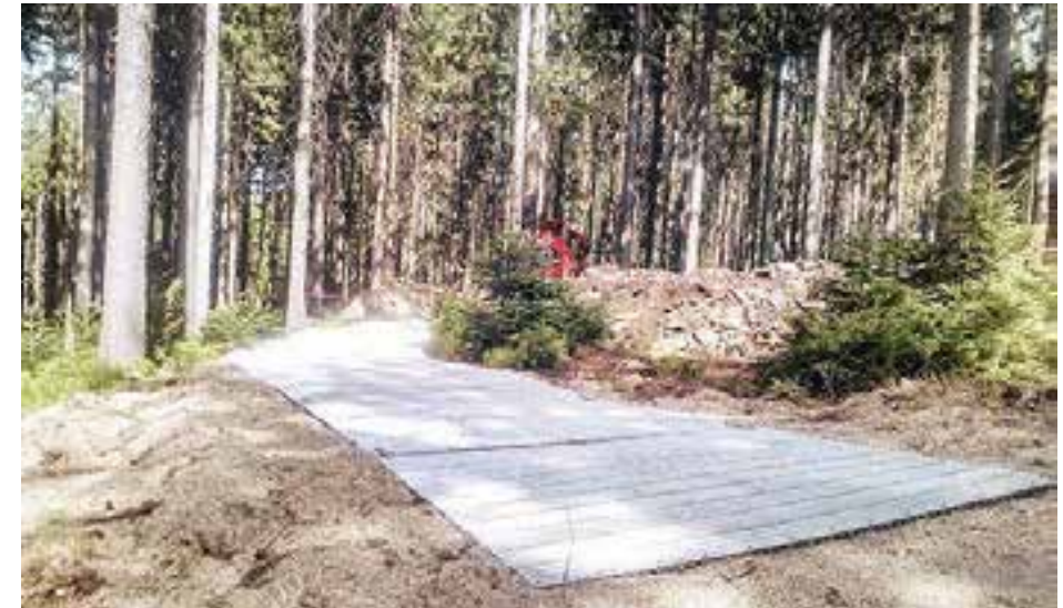
Deck Mat/Construction Access Road
